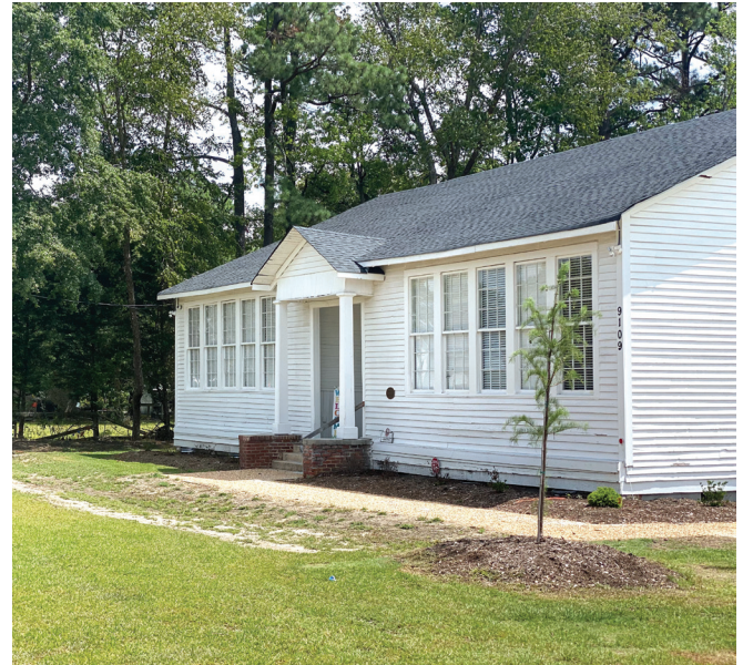
Exterior of the renovated Panther Branch Rosenwald School.
